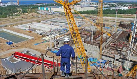
In frameworks of the project, Kompakt, JSC carries out works for concrete pouring of reactor building structures with transport gate, control building and steam chamber building, as well as the complex of works at the second power unit: bed drainage, concrete prepartion and concrete pouring of structures (reactor building with transport gate, control building and steam chamber building).
